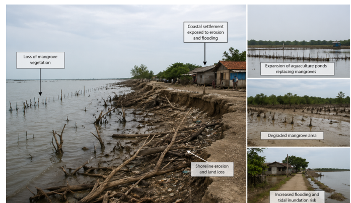
Figure 3. Field condition of Muara Gembong coastal area showing mangrove degradation and coastal vulnerability (documented by the authors, 2026).
