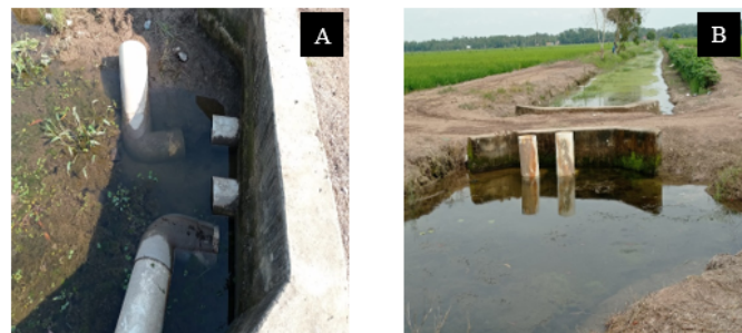
Figure 5. Water gate operation when open (A), sluice gate operation when closed (B)
