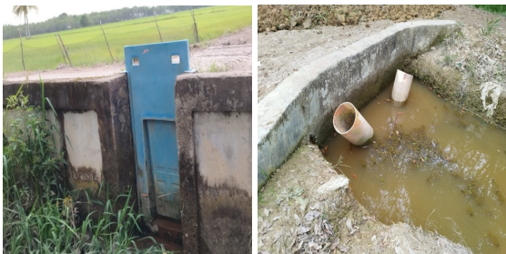
Figure 3. State of valve gate in the field (A), State of gooseneck gate in the field (B)
